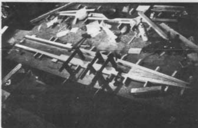
A very good method for making the 680 beams, using a table jig, with wooden blocks holding the timber flanges in the right shape. Photo from Leo Peters, who is building his 680 at Kalamazoo, U.S.A.
